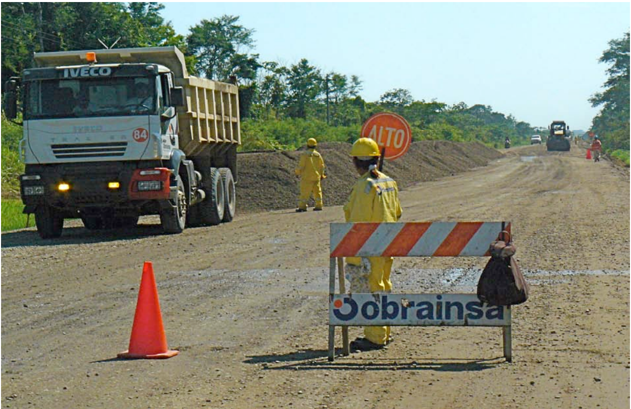
The Inter-Oceanic under construction to the west of Puerto Maldonado. 09 November 2008.
